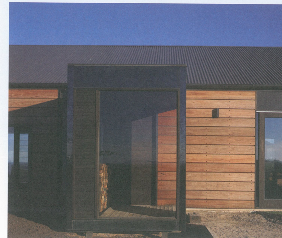
3 The varying size and apparently random arrangement of door and window openings is inspired by local agricultural buildings.
