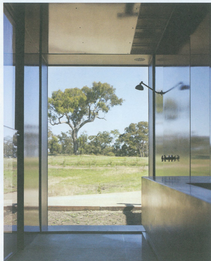
2 The use of mild steel cladding instead of tiles gives a strong industrial aesthetic to the bathroom, completed with concrete benches, vintage taps and a yellow rubber floor.
